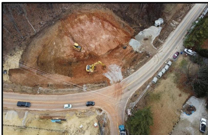
Reconstruction of two county road intersections at East Rock Creek and Spring Forest was also included. These two projects involved major grading operations including a 20-foot cut and a 30-foot fill. This project opened to traffic in May 2023 and cost an estimated \$5.2 million plus utility relocation costs.
