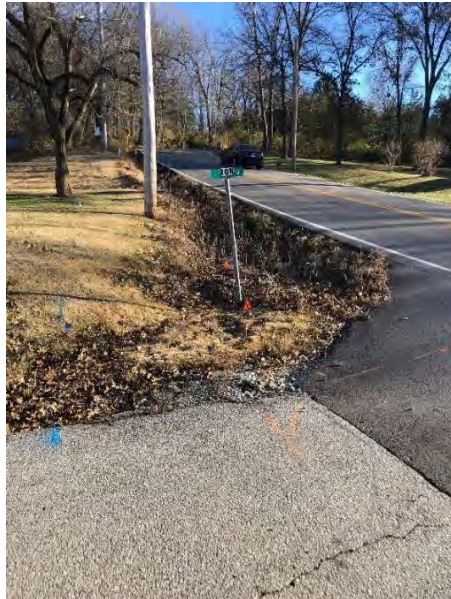
PHOTO 5: EDGE DROP OFF ON OUTSIDE OF CURVE
