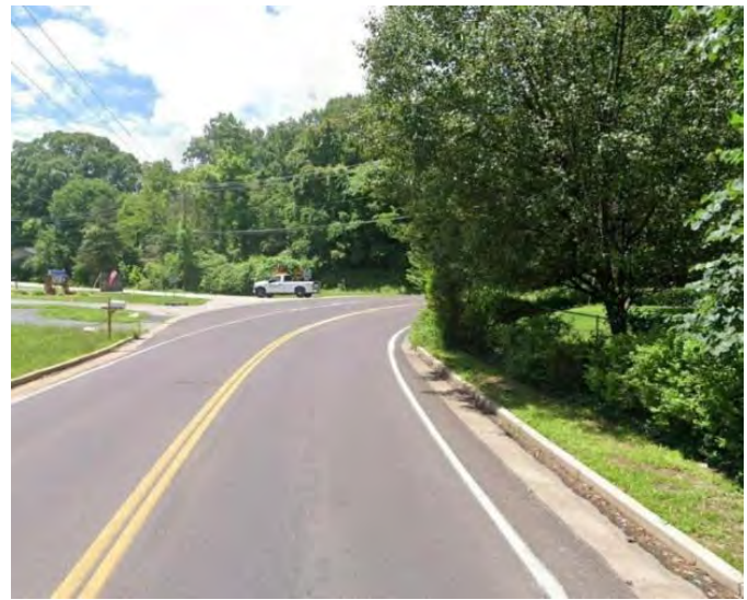
PHOTO 8: VEGETATION BLOCKING SIGHT DISTANCE ON INSIDE OF CURVE
