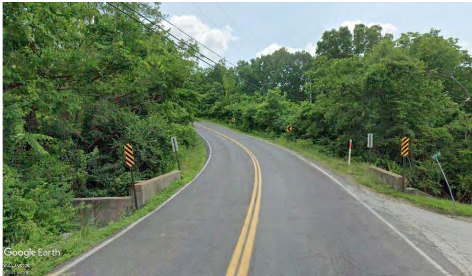
PHOTO 3: CULVERT HEADWALLS ADJACENT TO ROADWAY
