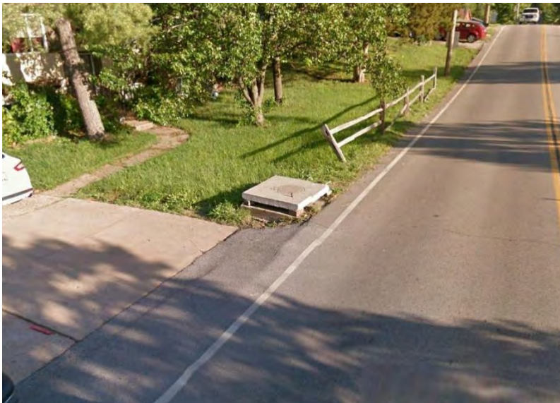
PHOTO 17 C: NON-TRAVERSABLE DRAINAGE STRUCTURE
