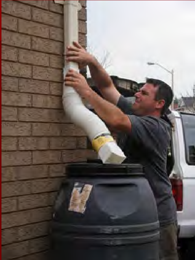
Downspout Disconnect
