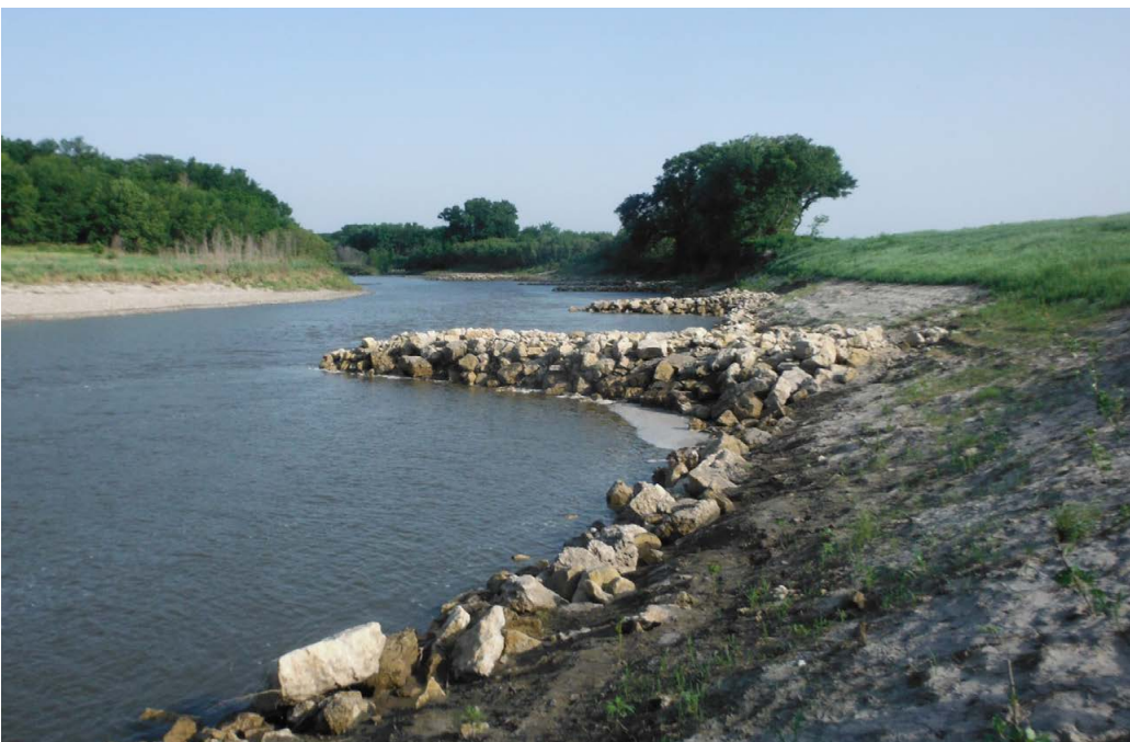
Recently constructed toe protection with bendway weirs.
