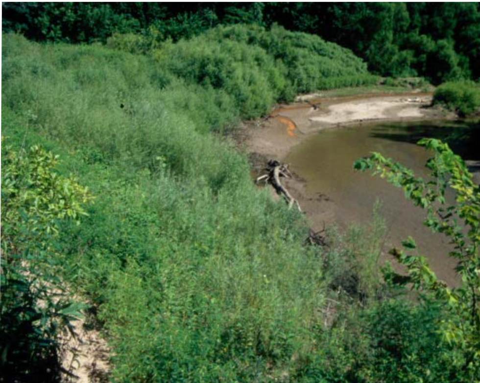
An eroding streambank with dormant willow stakes and the same streambank below after vegetation has started to grow.
