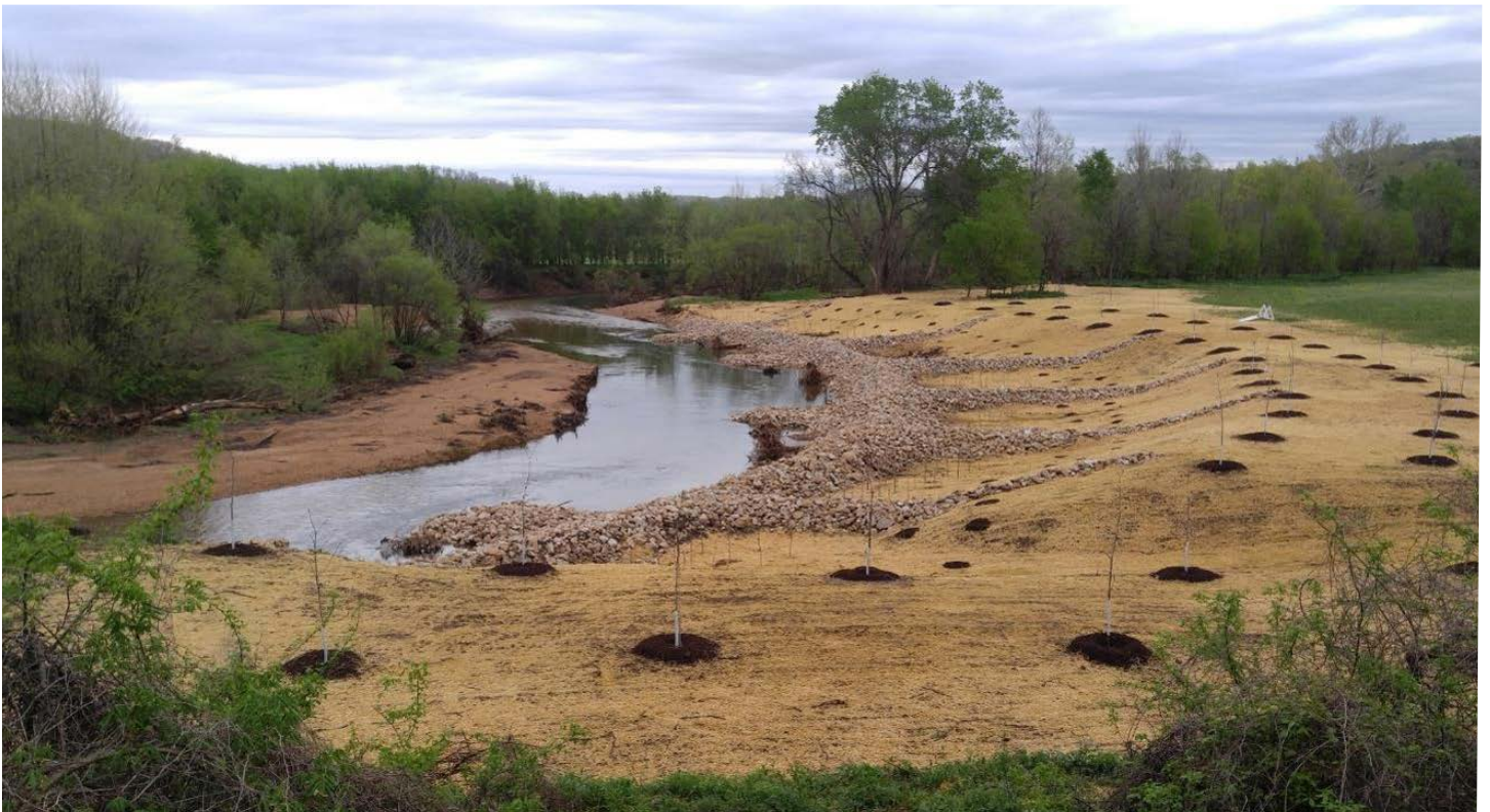
The same bank as above after re-sloping and LPSTP.
