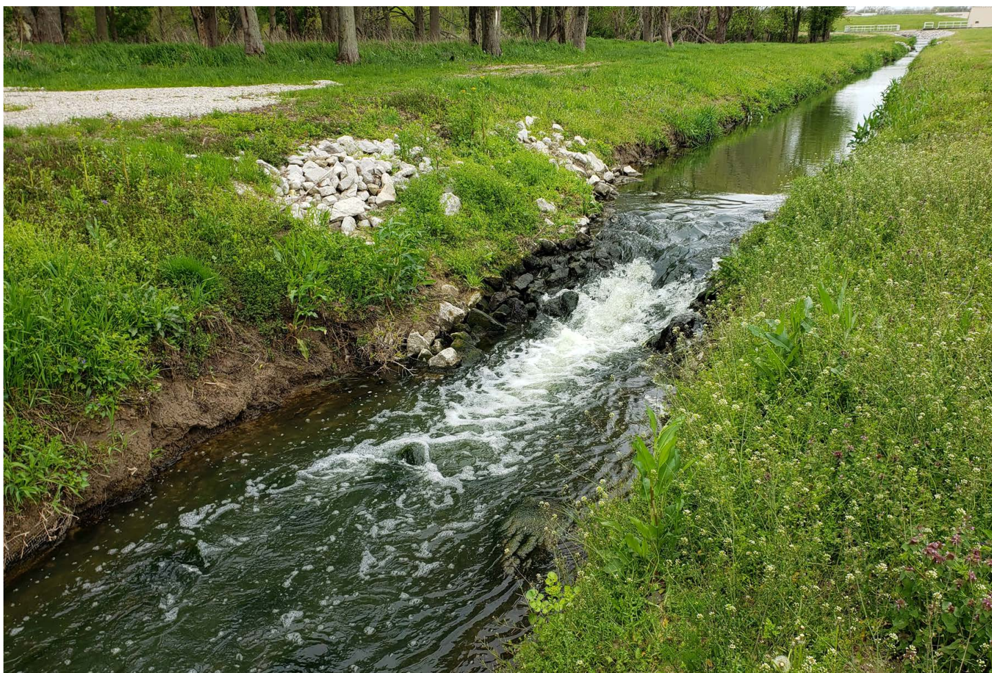
Rock grade control structure in a small channel.
