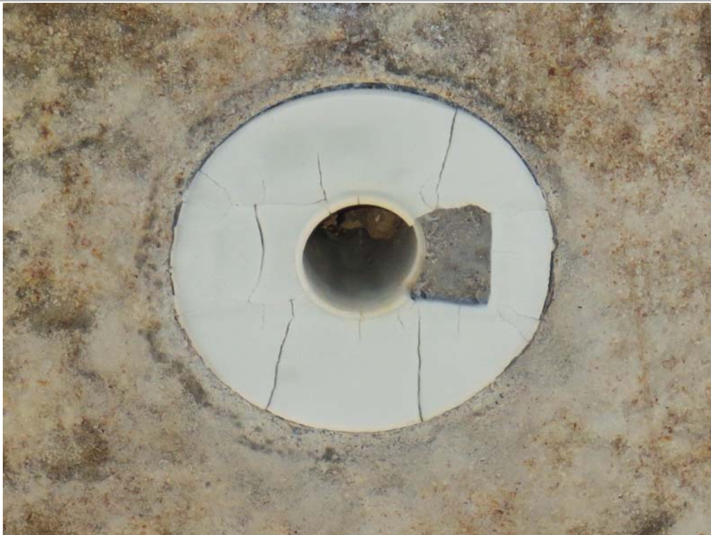
Photo: 4 View of torus-shaped drain outlets located on the underside of the bridge deck. The drain outlets were not readily accessible for testing.
