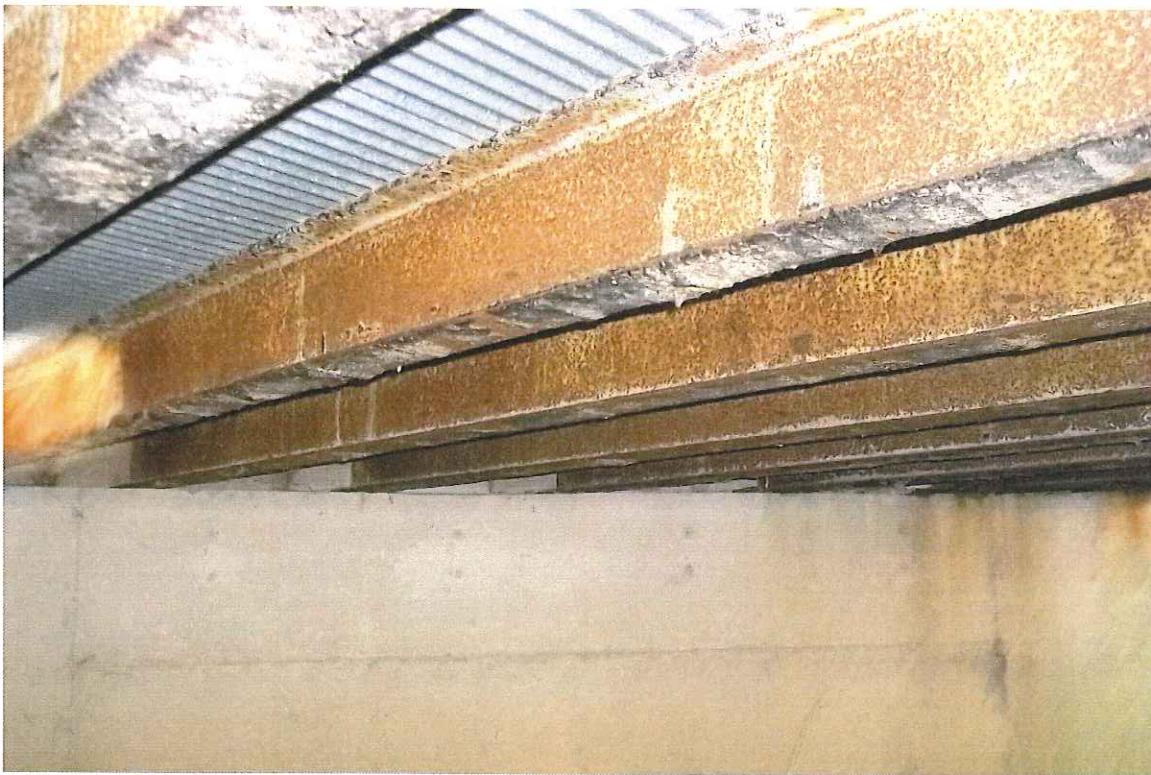
Photograph 3 ▲ - View of north half of bridge substructure. Note traces of silver paint on I-beams and tar-like potential ACM on underside of I-beam.
