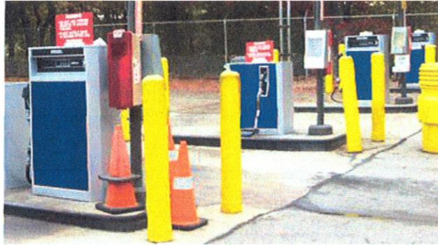
All remote dispensers include a satellite connection as standard so that they can be piped to an opposing satellite dispenser for the convenient fueling of truck saddle tanks or vehicles positioned with their tank on the opposite side.
